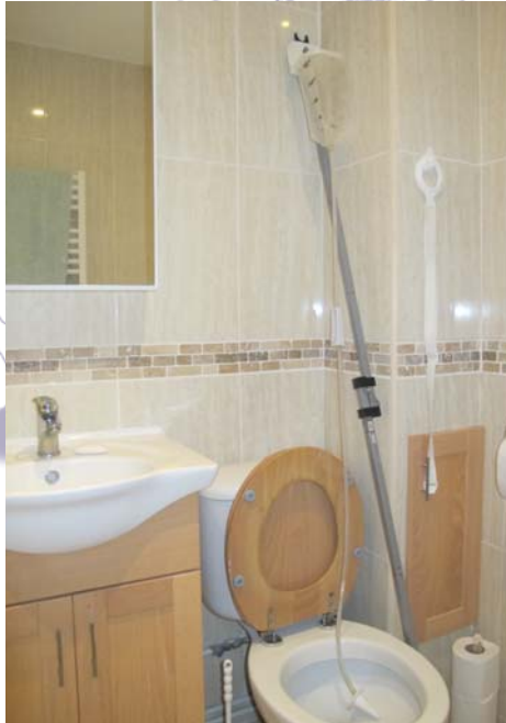
The typical bathroom set up
